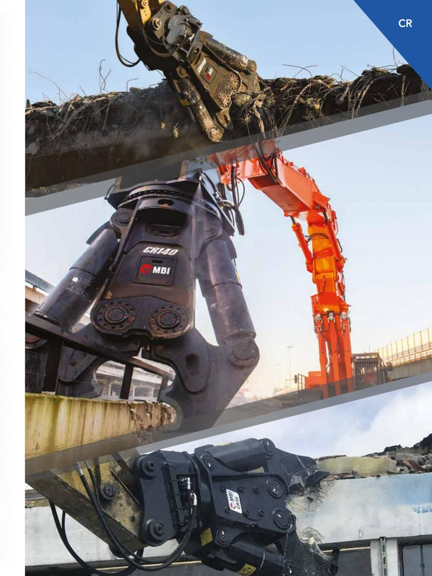
The **specific tooth profile**, studied to remain sharp despite wear, maximizes penetration.
